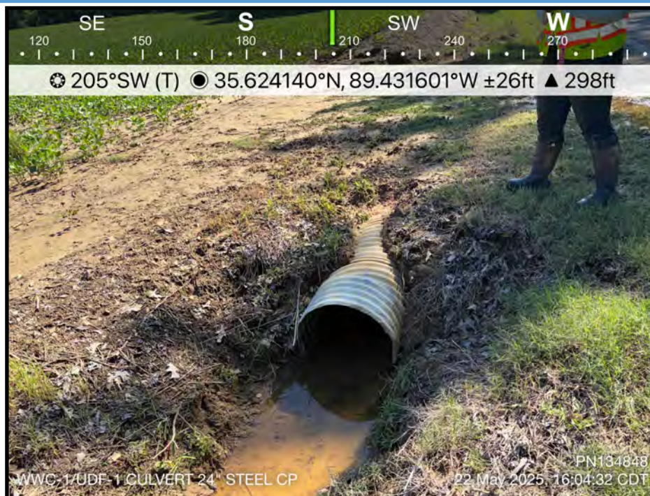
Photo 4: WWC-1/UDF-1 Culvert 24" Steel CP facing upgradient
